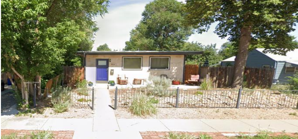
View of the property to the east, looking east.
