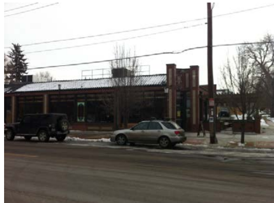
View from 28 th Ave. of the subject property.
