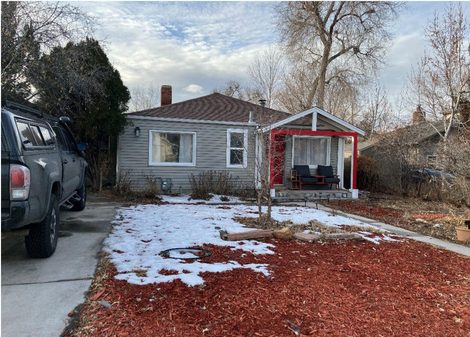
1. Front view of the subject property, looking west on S. Kearney Street.
