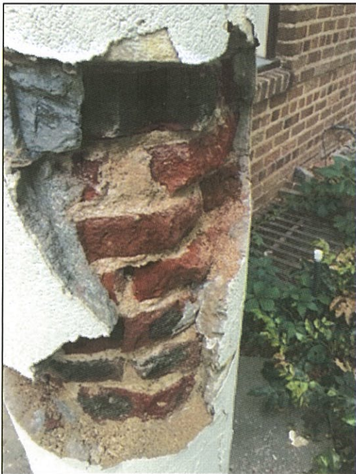
Brick column supporting front porch, photo taken during recent repairs (Source: Owner)
