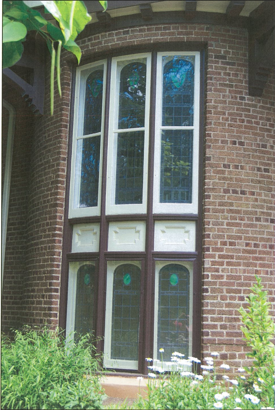
Stained glass on southwest corner
