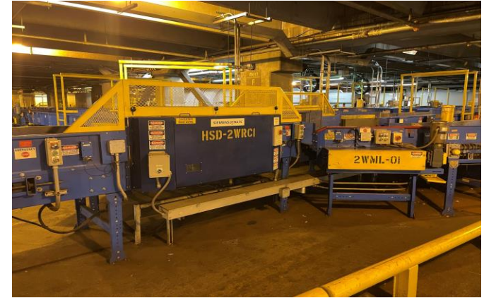
DEN TML Level 3 – Existing High-Speed Diverter
