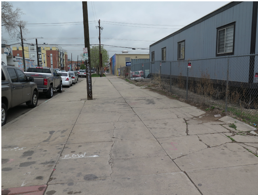
Lots of cracking in concrete sidewalk
