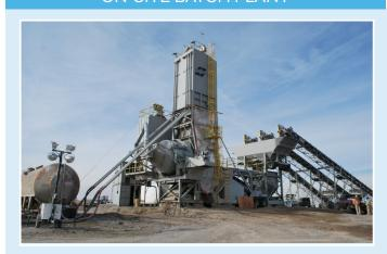
As of 2021, Flatiron's on-site batch plant carries six mix designs used extensively for our ongoing work at the airport.
