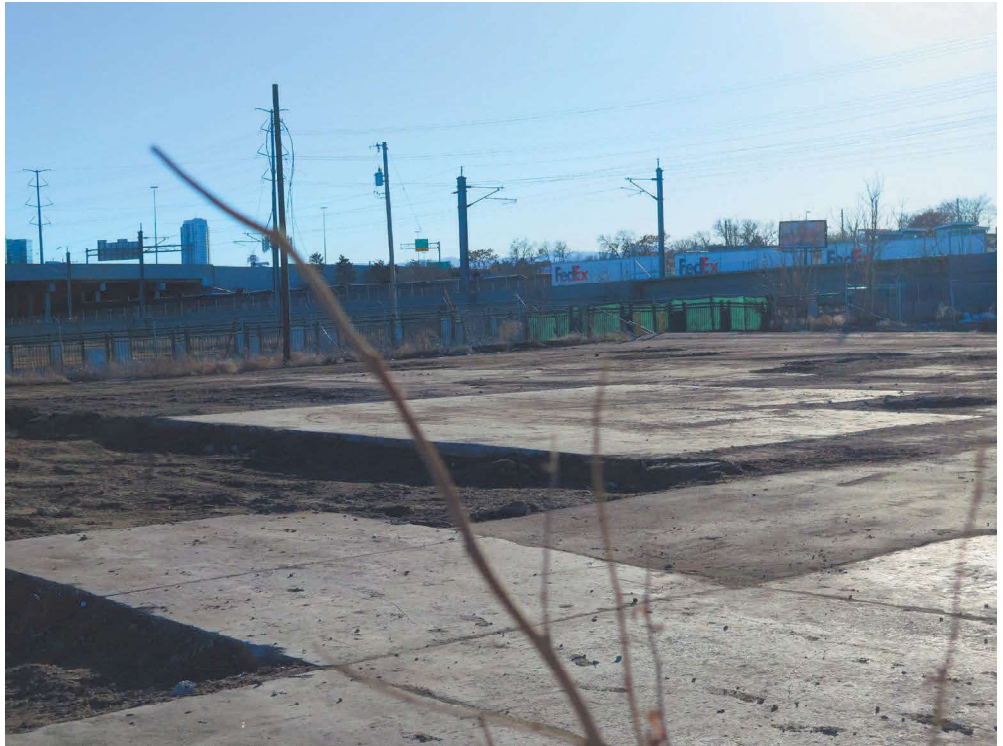
Concrete slabs with uneven grading
