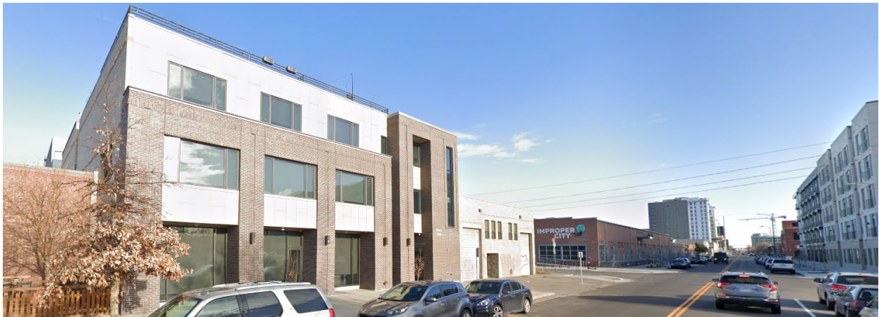
Northeast – view of the building to the Northeast, looking north.
