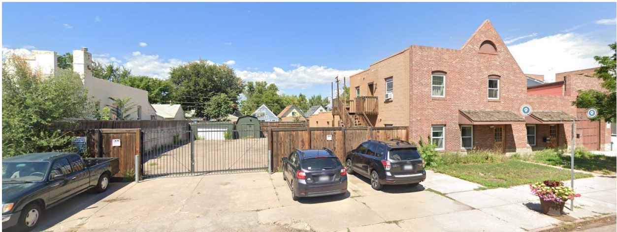
View of 1253 South Pearl Street, looking west (Source: Google Maps)
