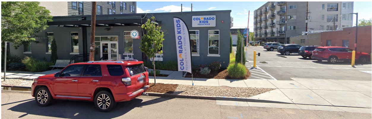
View of the 1-story commercial property along South Pearl Street, looking east (Source: Google Maps)
