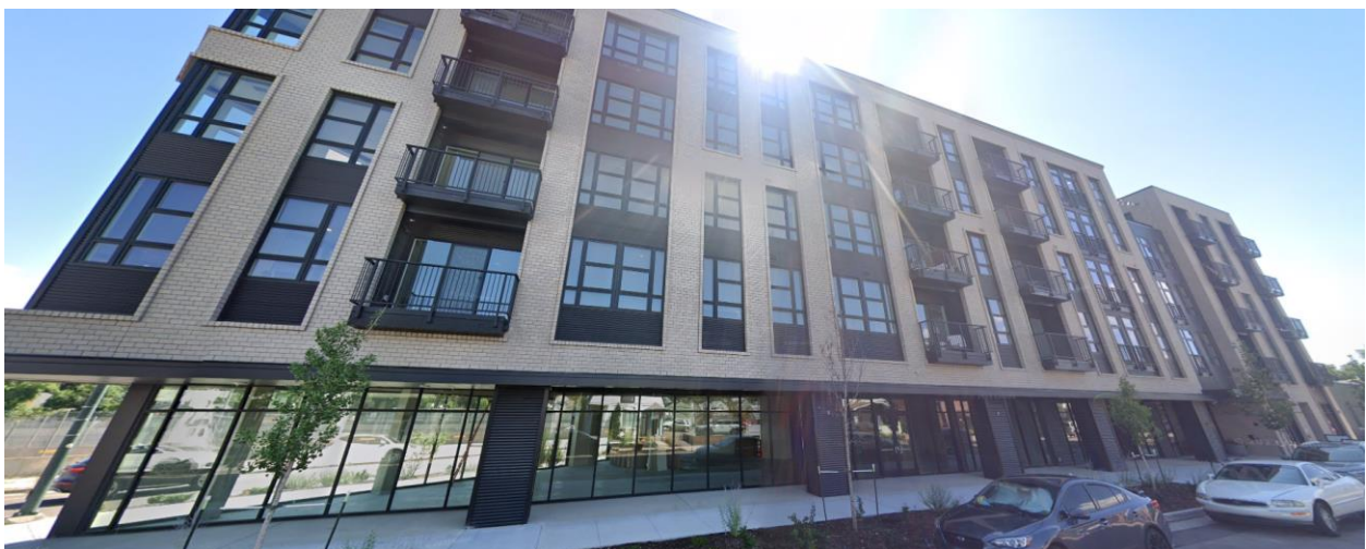
View of the 5-story mixed-use property along South Pearl Street, looking east (Source: Google Maps)
