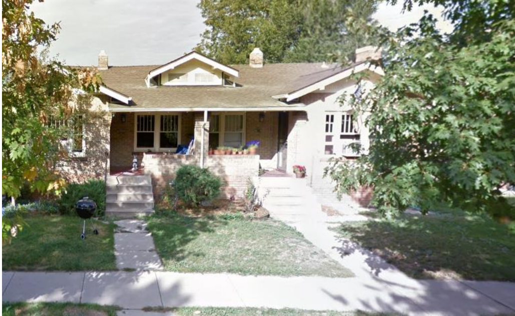
East - View of the property to the east, looking west.
