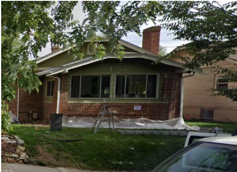
Subject Property - View of 560 South Emerson Street, looking east.
