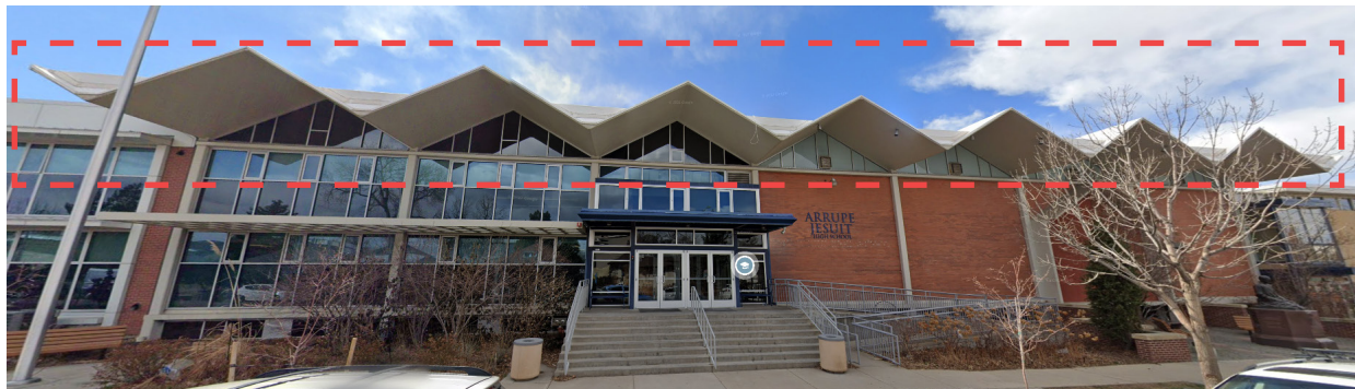
Figure 1-2 Existing folded plate roof (Source: Google Maps)
