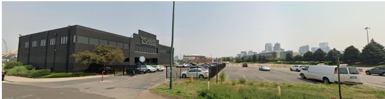
View of the subject property from 5 th Street, looking northeast.
