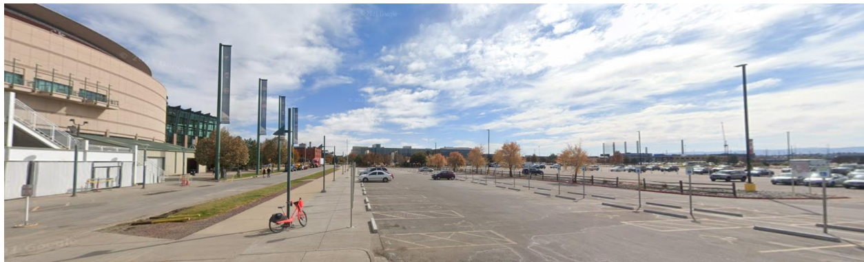
View of Ball Arena and the surrounding parking from the Ball Arena/Elitch Gardens train station, looking southeast.
