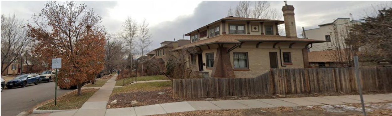
View of the 2-story single-unit residential property to the south of the Center along Stuart Street, looking south.
