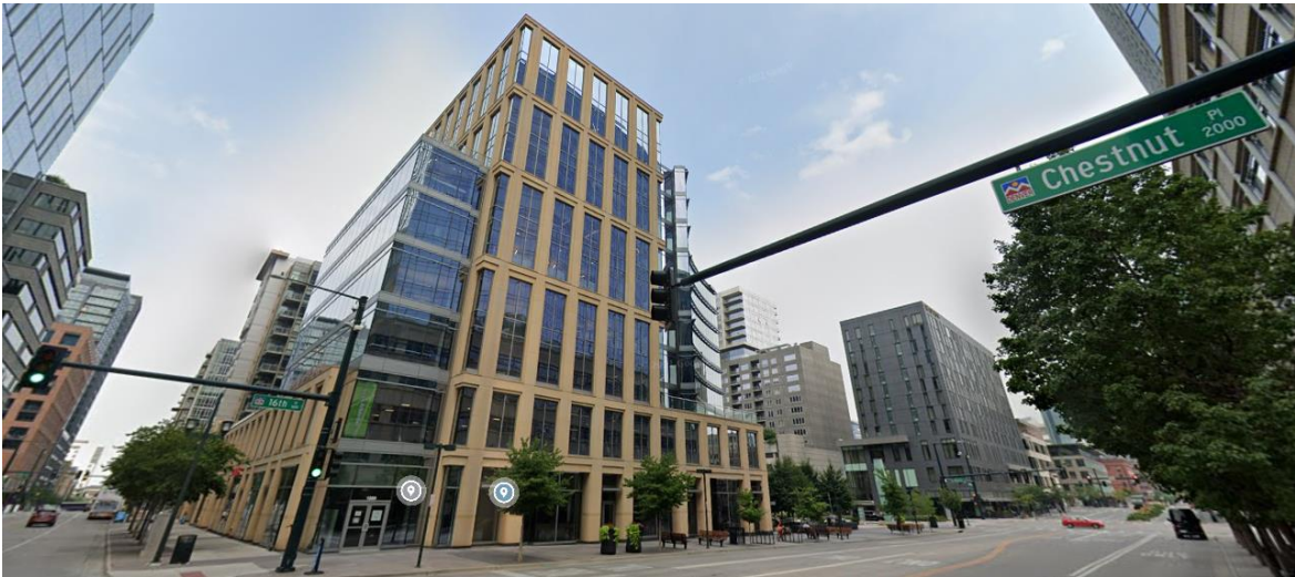
The property to the south across Chestnut Place at the intersection with 16 th Street, facing east.
