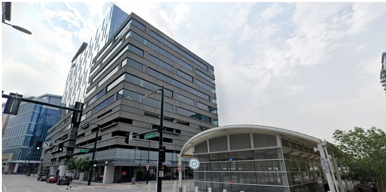
The subject property with the 11-story portion in the foreground, from Chestnut Place looking west.
