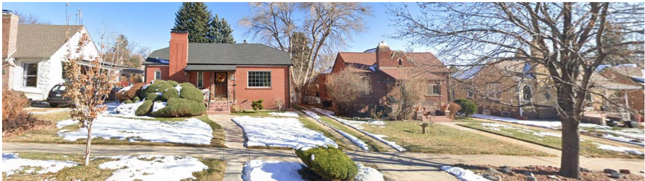
View of the 1-story residential properties to the east of the Center along Stuart Street, looking east.
