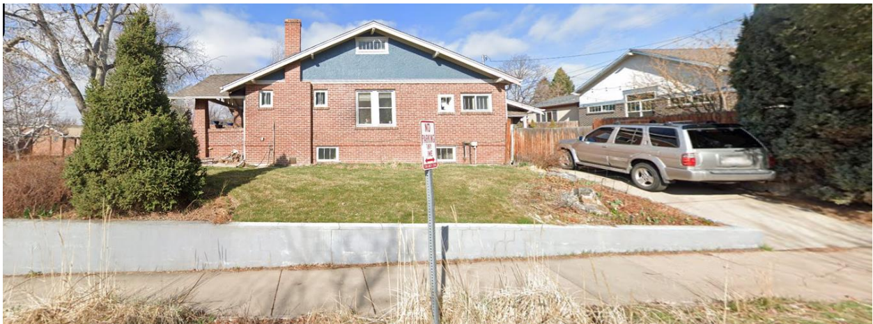
View of the 1-story single-unit residential to the west of the Center, looking west.
