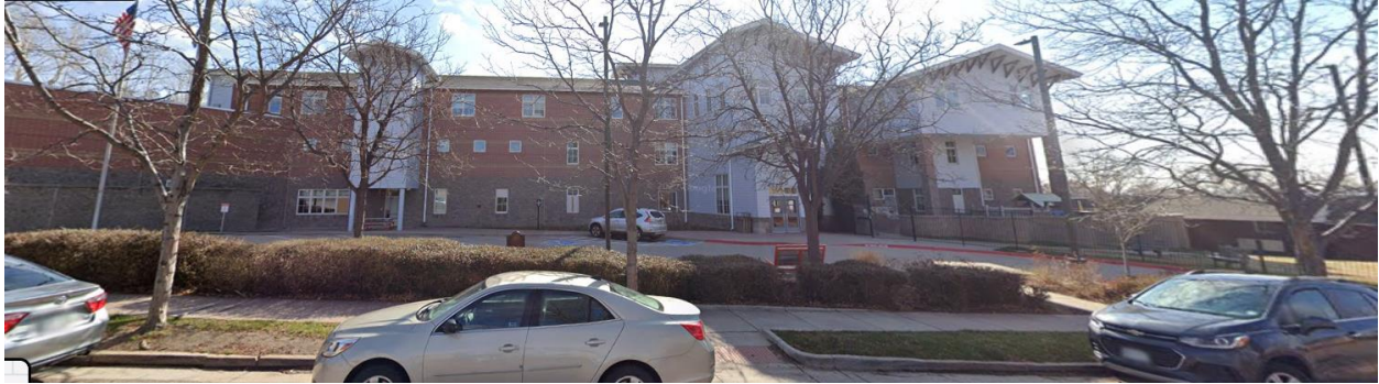
View of the main Center building located along Tennyson Street, looking east.
