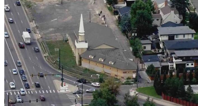
Photo taken pre-demolition
