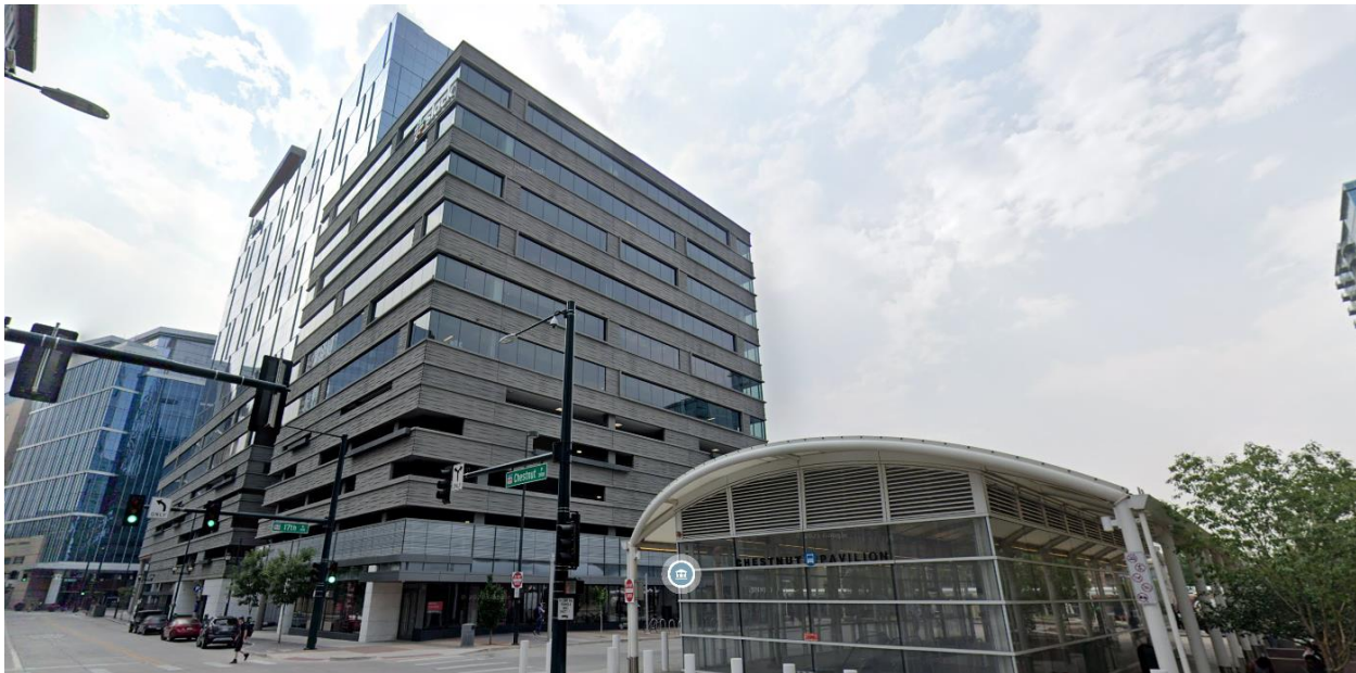
The subject property with the 11-story portion in the foreground, from Chestnut Place looking west.
