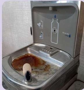
Water fountain with dirty still water
