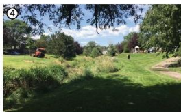
Example: 140' wide Weir Gulch greenway with 4:1 slopes, trail and natural channel
