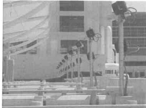
Upon removal of the media (ticket or credit card), the Entry Terminal signals the gate to open. The vehicle activation of the gate loop causes the LPR system to begin image recording. The loss of the vehicle detection on the gate loop disables the image recording. During the image capture process the LPR system digitizes several images of the vehicle's rear, selects the optimal image, reads the license plate and determines a confidence factor for each license plate read.
