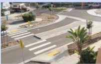
Median and pedestrian crossing islands near a roundabout. Source: www.pedbikeimages.org / Dan Burden
