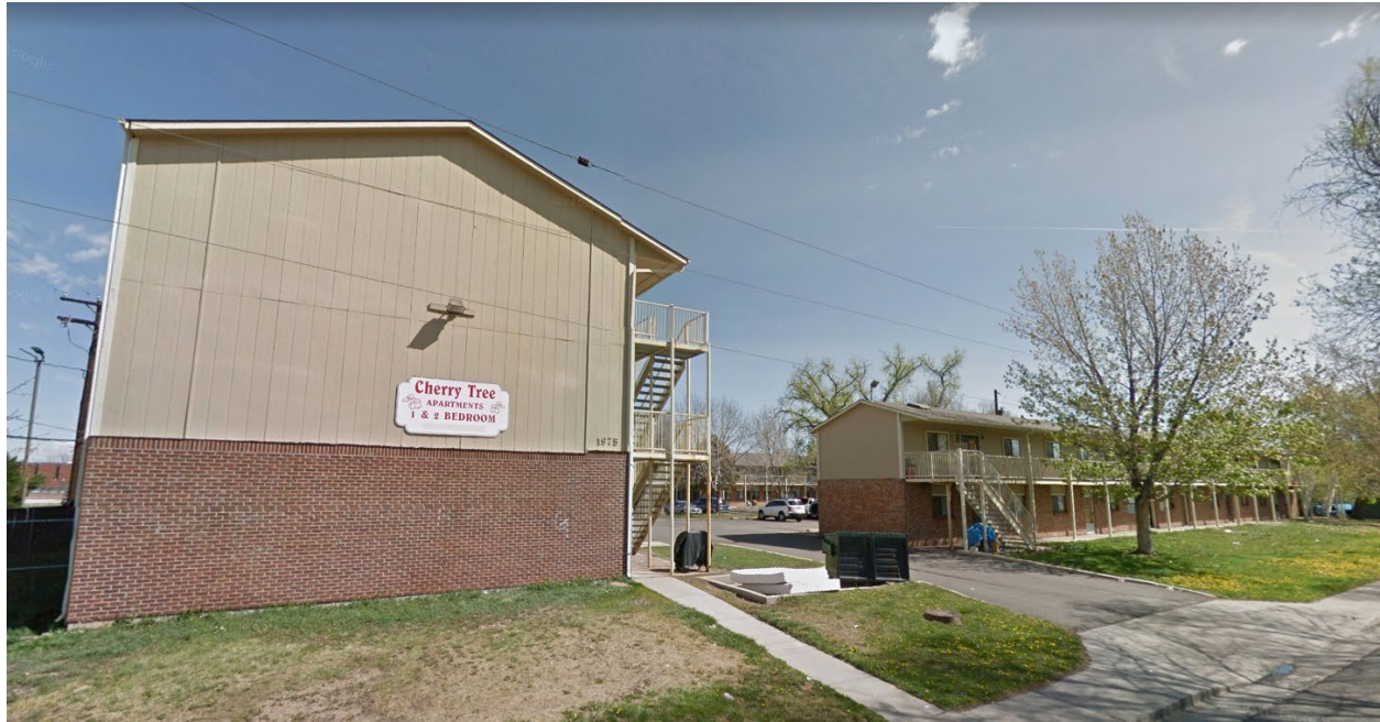
View of subject site on W. Asbury Avenue, looking northeast.
