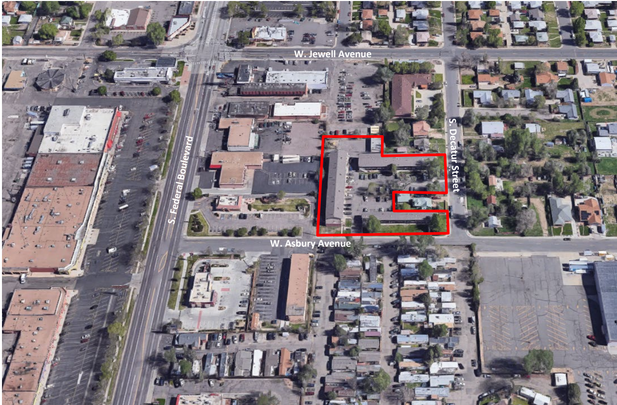
Aerial view of subject property, looking north.
