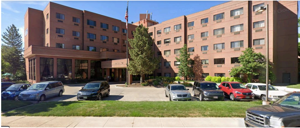
East of the subject property, facing north from Yale Avenue
