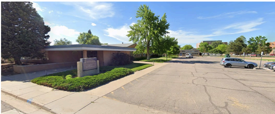
Subject property, facing north from Yale Avenue
