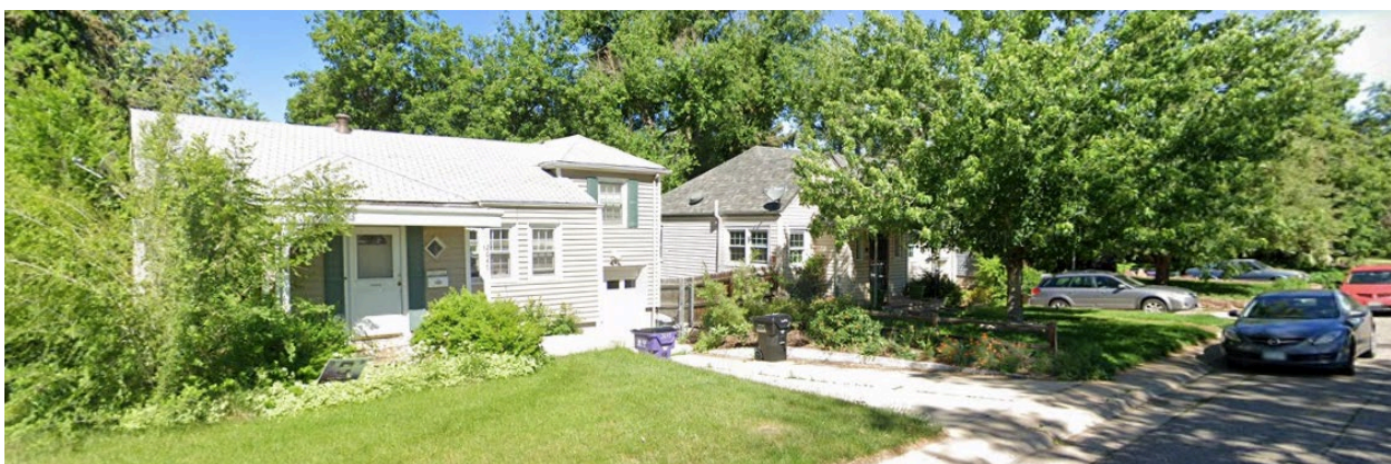
West of the subject property, facing west from S Clarkson Street
