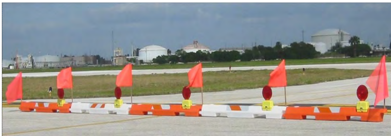
Figure 2-8. Interlocking Barricades
