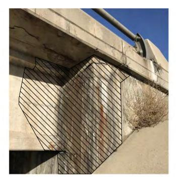
ABUTMENT 12 - ABUTMENT, GIRDER AND WINGWALL SPALLS SPALLS
