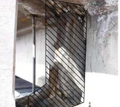
PIER 5 - SOUTH END OF DIAPHRAGM SPALL
