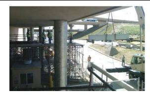
Material including 40' long sections of guiderails, train switches and sections of the center turntable switch were craned into Level 4 of DIA's main terminal through an 8' x 8' opening cut through the precast and masonry walls.
