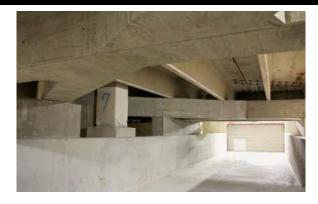
New concrete beams and walls were installed in Level 3 tight to the existing 30" deep twin tees resulting in limited headroom above the formwork creating quality and safety challenges.
