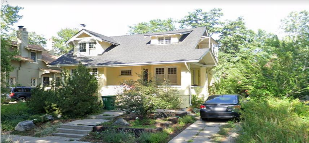
View of subject property looking east.
