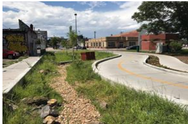
Green Infrastructure bioretention at 21st/Broadway
