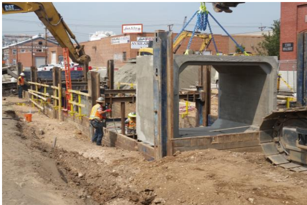
Large box culvert installation in RINO/Five Points
